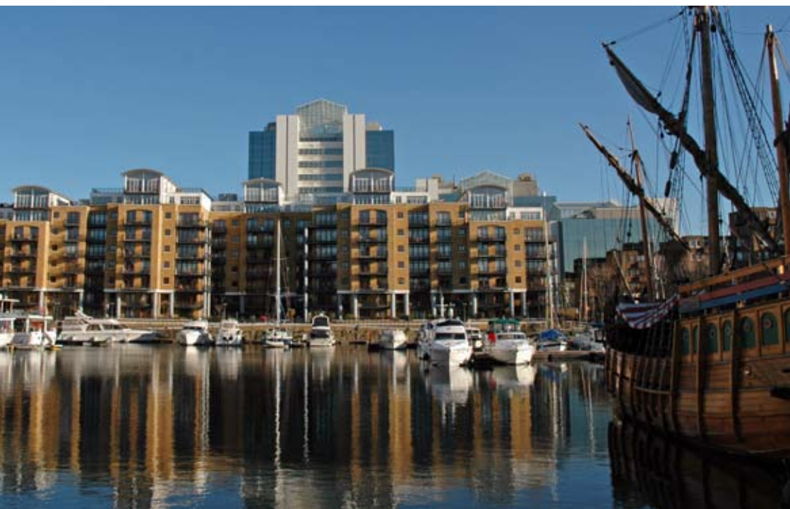
Handelsbanken's London operations have been located in Trinity Tower since 1997. As of 1 January 2008, this is where the regional head office for Southern Great Britain is situated.
